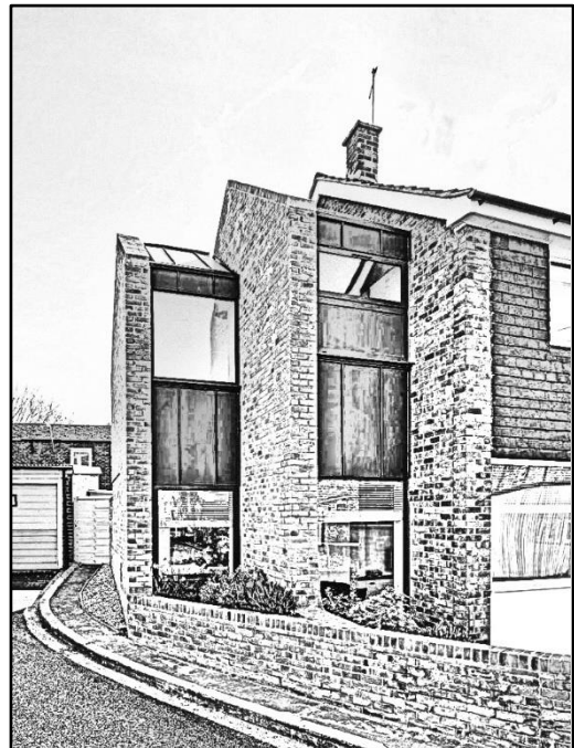
Figure 1.12b - Successful side extension that incorporates a mix of contemporary and matching external materials with larger windows
