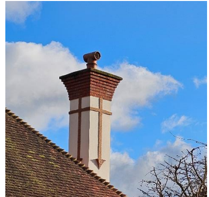
Figure 4.30a: Contemporary chimney with brick detailing
