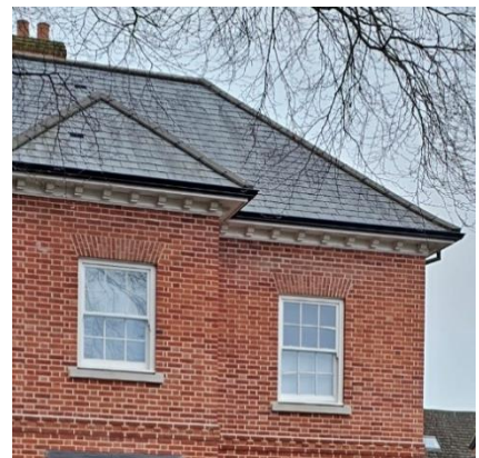
Figure 4.30b: Decorative stringer course, brick bond and bracketed cornice
