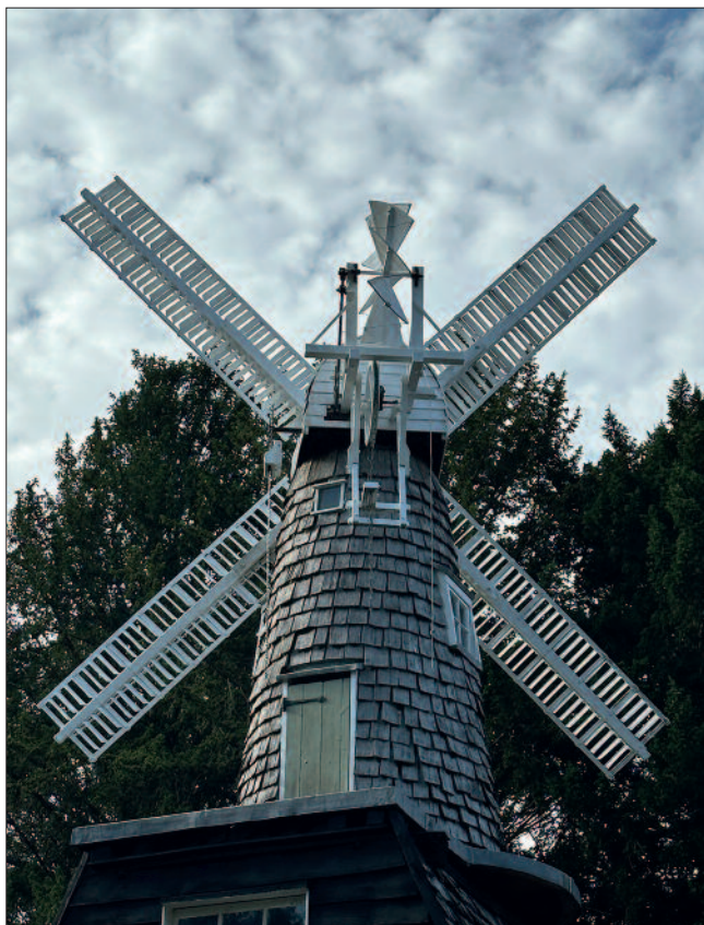
Two views of the tower in 2024.
