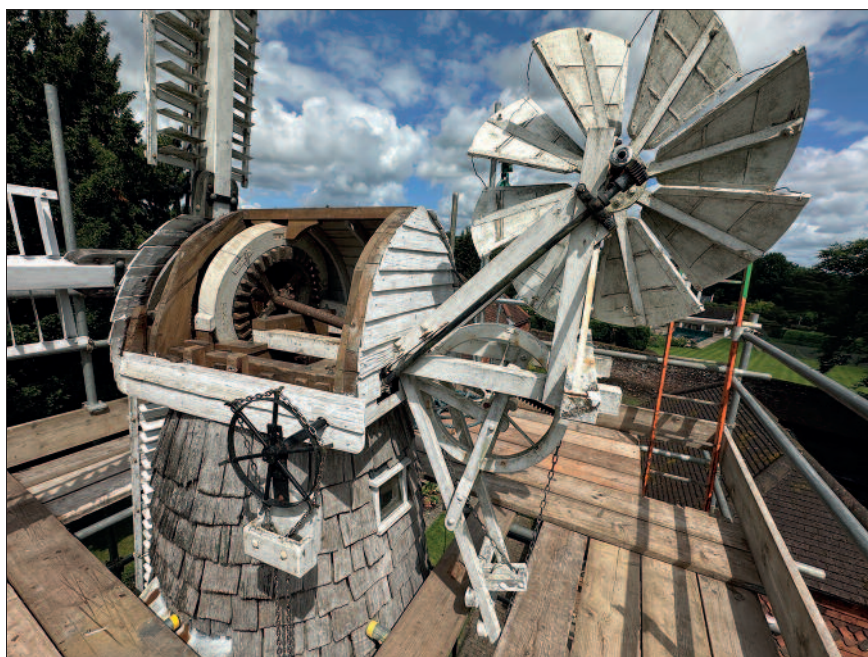
The cap undergoing maintenance in 2024, before painting.
